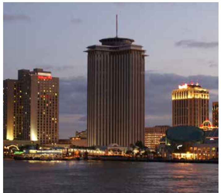
Figure 1. A view of the World Trade Center. The building is currently being renovated into a Four Seasons Hotel. Source: Wiki Images.
